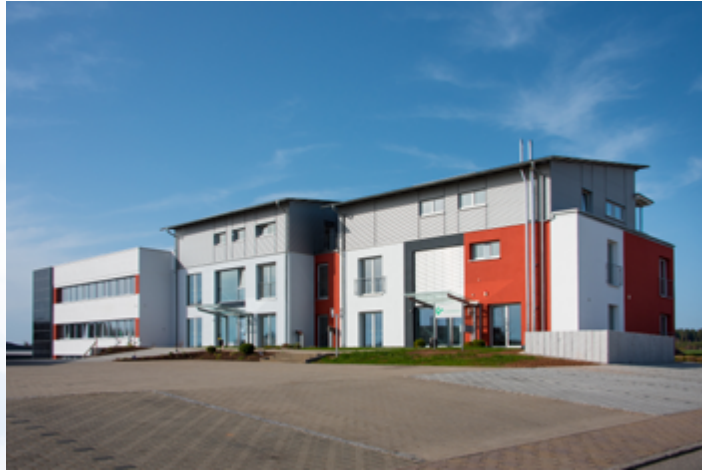
(CS-Instruments head office and production facility in Germany)
